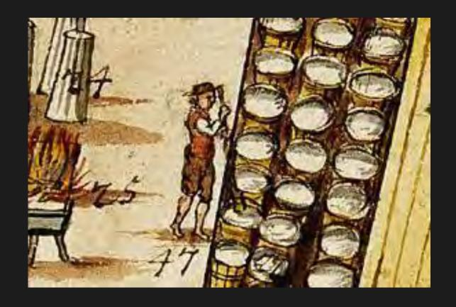
The next step was to stamp the hot salt in moulds. Those standardised wooden moulds had the form of a cone.
